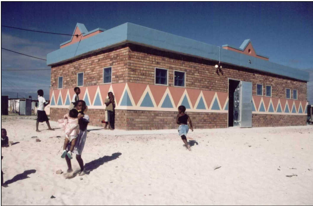
Figure 9: Completed Chamber in Khayelitsha
