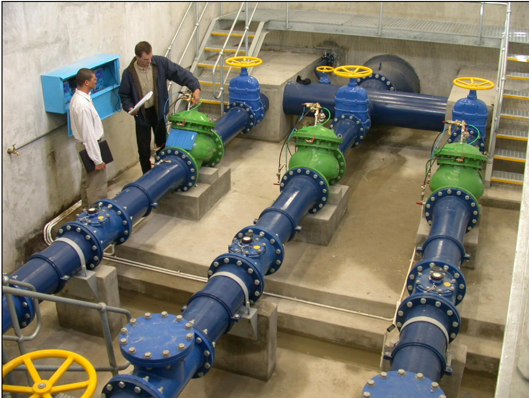
Figure 5: Internal View of a Portion of the 1065 mm diameter Chamber
